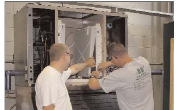
In the hands-on lab at Ferris State University's Granger Center, (left to right) Jason Alder and Tom Pennington troubleshoot a problem with a commercial ice machine.
