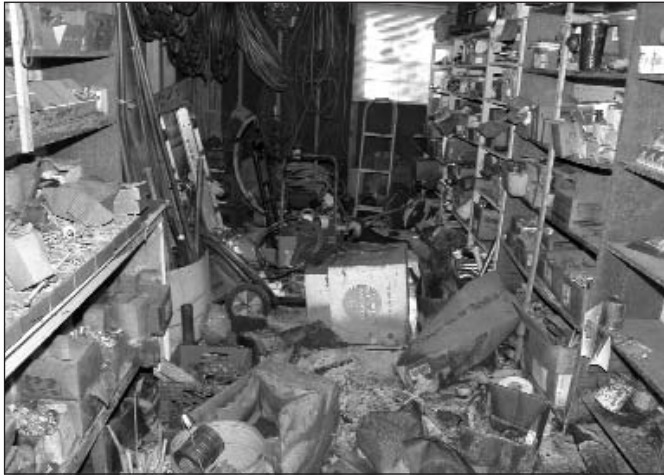
The flood wreaked its own brand of havoc in this parts storage room at Baudier Mechanical Contractors in St. Bernard Parish.
