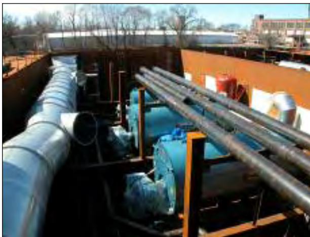
Boilers and other heavy components had to be set in the hold deck before erection of the top deck.
