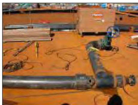
Large fabricated pipe waits to be lifted and set into the ship's hold.
